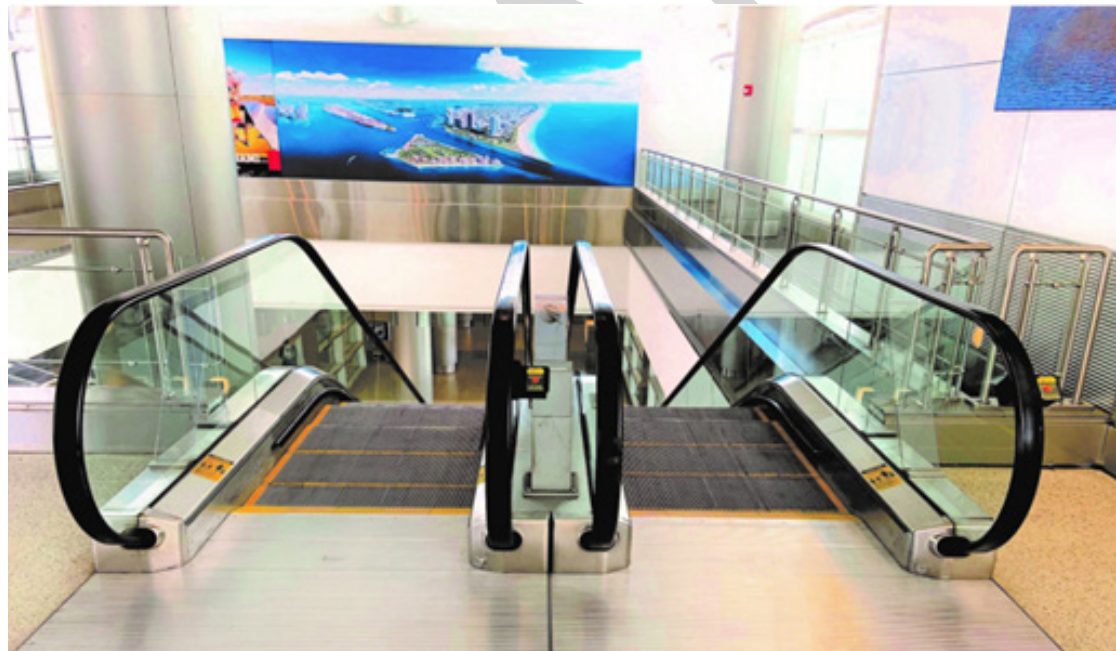
Escalators at MIA
