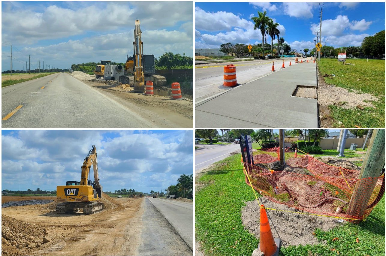
SR 9336/SW 192 Avenue from SW 376 Street to SW 344 Street Construction
