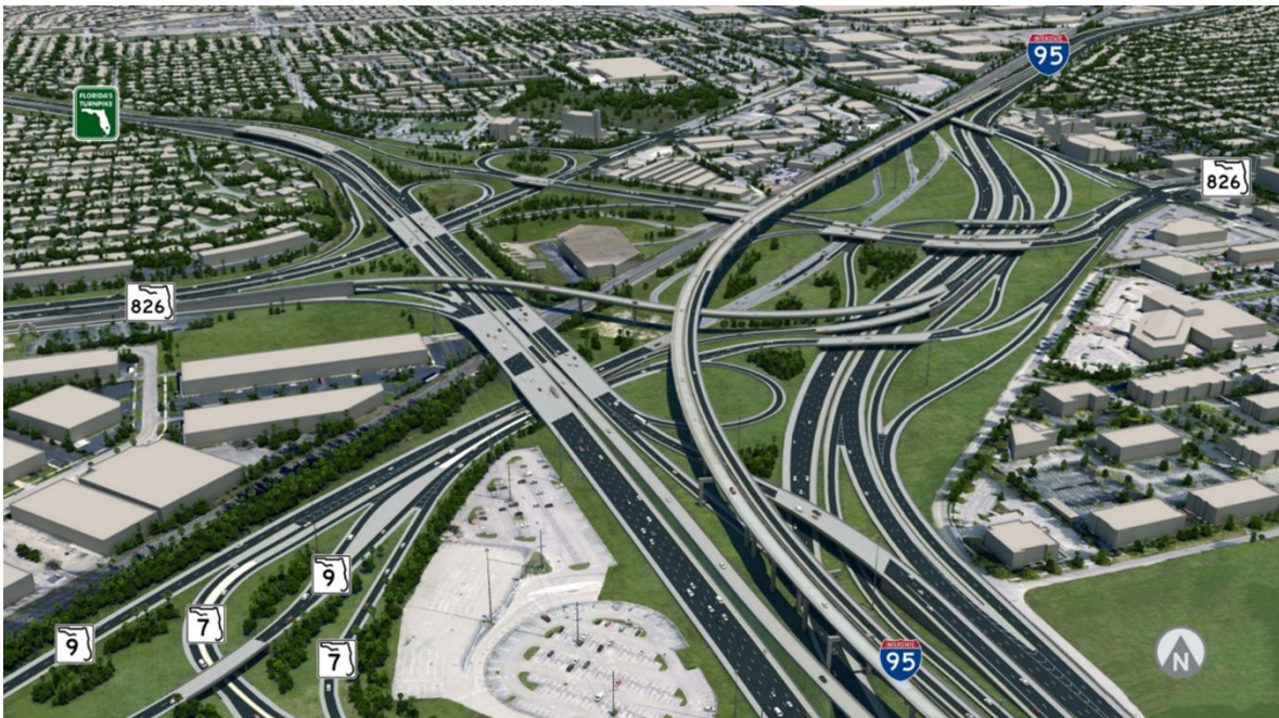
Golden Glades Interchange Improvements
