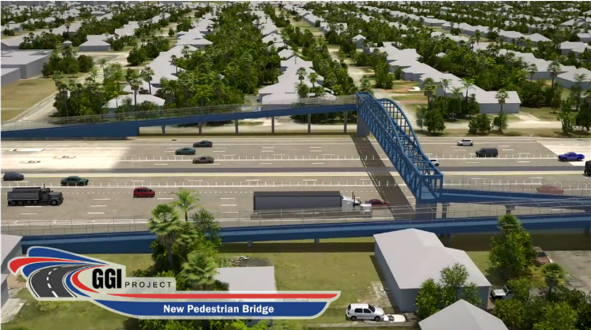
Golden Glades New Pedestrian Bridge
