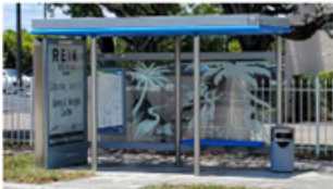
Shelter with an advertising panel
