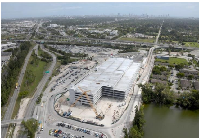
Construction Progress – Spring 2020
