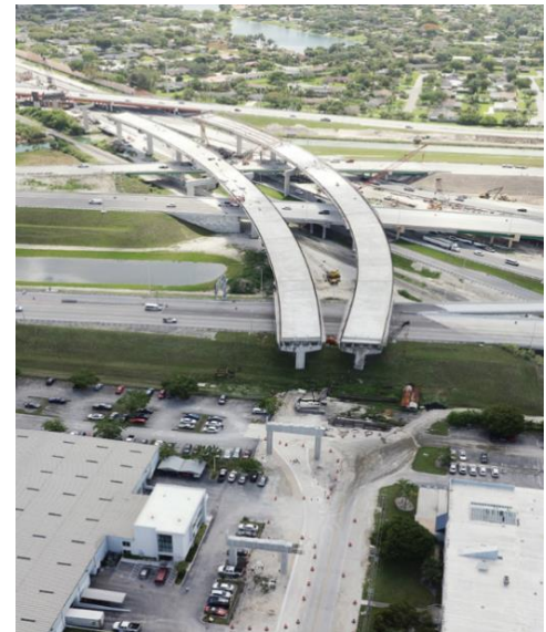
SR 874 Northbound/Southbound Connector Bridges to SR 874
