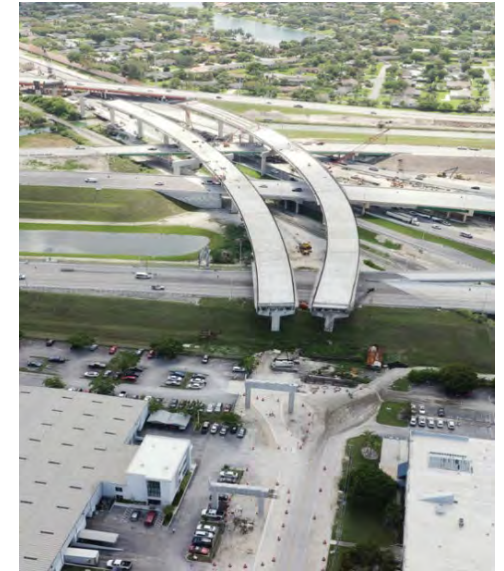
SR 874 NORTHBOUND/SOUTHBOUND CONNECTOR BRIDGES TO SR 874
