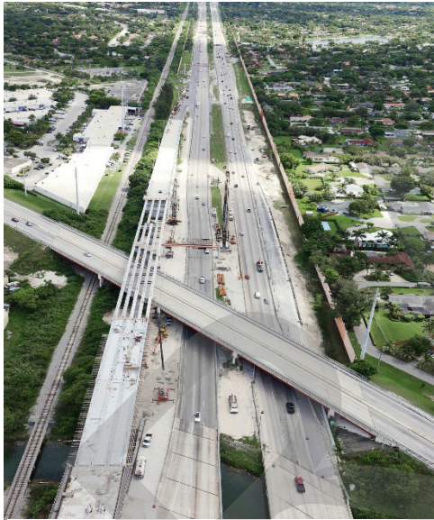
SR 874 Southbound Connector Looking North
