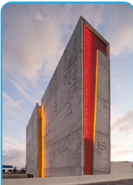
Port of Miami Tunnel Landmark
